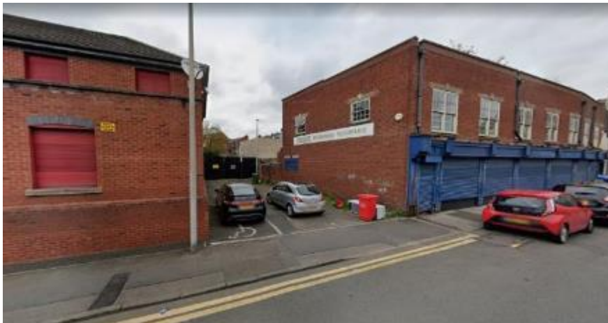
Figure 69 Gap site Russell Street. Google Streetview.
