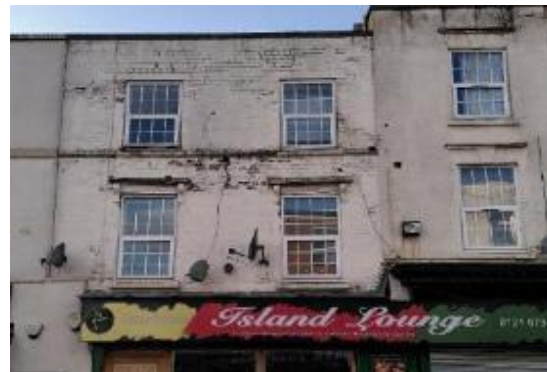
Figure 19 Rendered and painted brickwork typical of 19th century frontages
