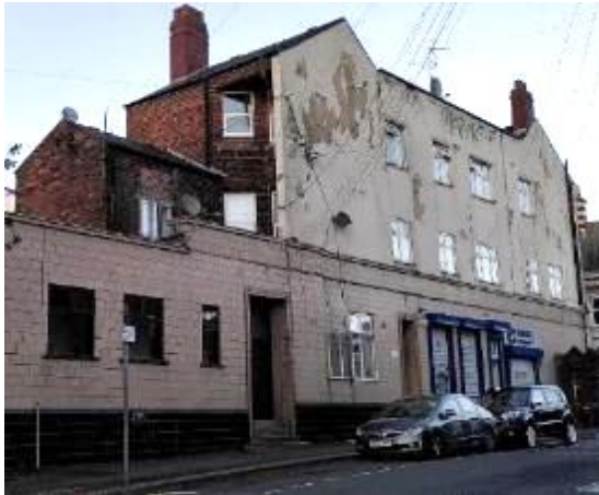
Figure 14 Former George Inn, side elevation viewed from The Shambles.
