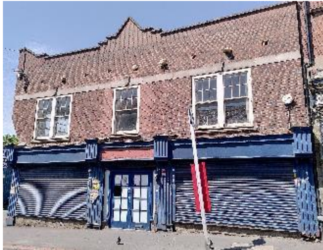
Figure 49 22-24 Lower High Street.
