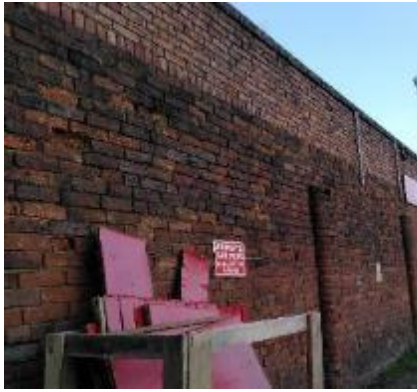
Figure 20 Wall, North of Shambles Car Park
