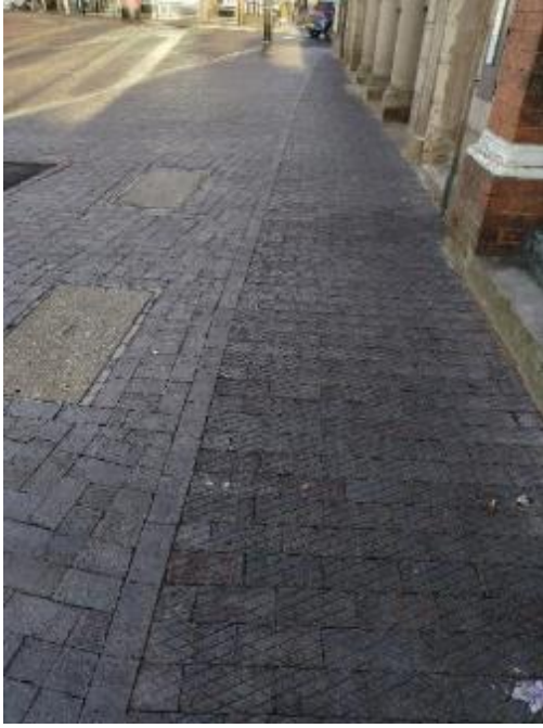
Figure 64 Blue diamond paving, Market Place
