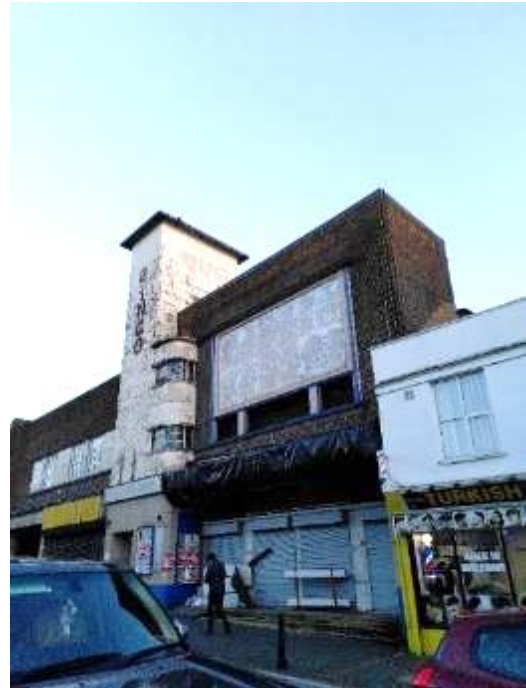
Figure 67 Locally listed former Gaumont Cinema, Walsall Street.
