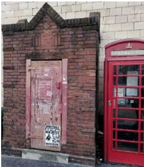
Figure 60 Police Box, Shambles.
