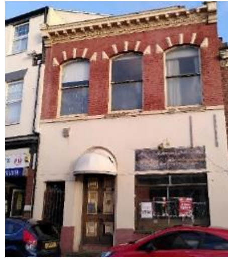
Figure 79 Poor quality signage, Lower High Street.
