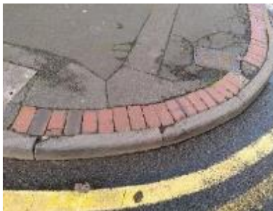
Figure 71 Paving Russell Street
