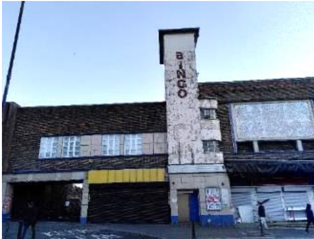
Figure 85 Former Cinema, Walsall Street.
