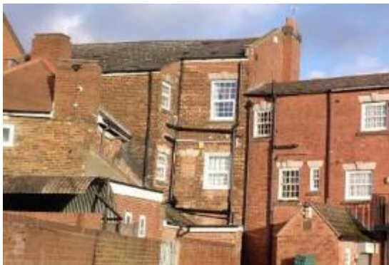
Figure 18 Rear of properties along Lower High Street
