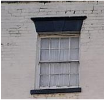
Figure 23 8/8 pane sash window, 32 Lower High Street
